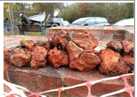
In the corner between the boiler house and chimney were a small number of loose clean bricks that had never been cemented. Some of the material came out in clay lumps.
