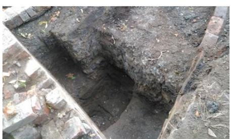
In the north east corner the wall has proved to be quite substantial with the brickwork being 18 courses deep. Although the shaft is 18<sup>th</sup> century, a theory is that the brickwork is 19<sup>th</sup> century, as Georgian bricks were smaller than Victorian bricks.
