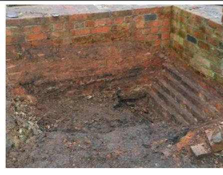
The corner between the boiler house and the chimney has been further excavated. While the bottom of the boiler house wall is straight and vertical, the bottom of the chimney wall expands in five stepped levels to provide a broader, solid base for the weight of the chimney.
