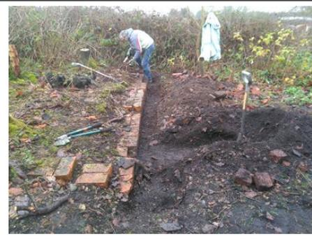
To the east of the cottage a brick pavement has been revealed, so far it is about a metre wide. As well as exposing the pavement the intention is to remove material from inside the house so as to reduce the one sided pressure on the walls.
