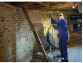
As soon as the first four sections of the central framework were free they were individually carried to the mill and carefully attached to the rope hoist.
