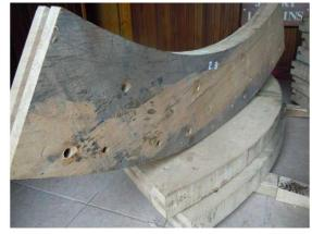
A side view of one of the rim timbers shows the range of holes drilled through it. Some were to hold the timbers together, then there were separate holes for the sections of cast iron teeth.
