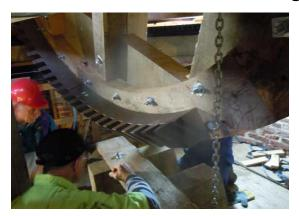
The cast iron teeth were bolted in position. It was heavy work lifting each segment up to the wheel and holding it in place.
