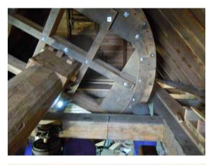
The team was again in full flow by 9am with multiple sockets and other tools needed to fit the 80 or so nuts that held the brake wheel components together.
