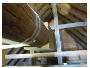
Concurrently the woodwork specialists were in the cap floor at the top of the mill fitting the first four central timbers onto the square part of the wind shaft.
