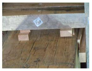
A close up of the wedges that ensured the brake wheel was positioned squarely on the wind shaft with an equidistant gap on each side.
