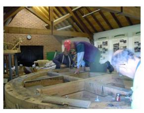
By 9am the team was already in full flow with multiple socket sets to undo the 80+ nuts on the bolts and studs that held the brake wheel components together.
