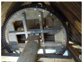
The almost finished brake wheel. After a year of work it is hard to believe that it is almost complete. The Trust spent £5,000 on materials and was very appreciative of a £1,500 grant from the Helen Jean Cope Trust towards the cost of the castings.
