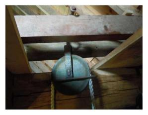
Hauling heavy timbers to the top of the mill required a substantial rope and pulley held in place on a solid structure on the cap floor.
