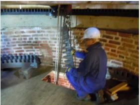
Cap Floor – the casting was carefully landed and manipulated to the storage area, two supports were used to spread the weight.
