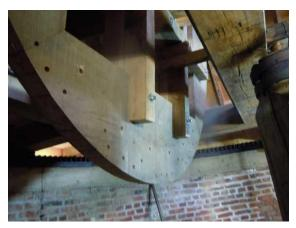
By the end of the day the brake wheel was looking good, with the central part of the outer rim having been fitted to the square inner framework.
