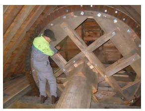
Final adjustments took place to ensure that the brake wheel was properly balanced. The whole project was a marvellous achievement by the volunteers. Very few new brake wheels are made and they are virtually all made by millwrights, joiners and contractors.
