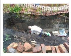
Underpinning the wall of the ventilation fan / winding drum pit. Cement blocks were inserted, some had to be cut to shape. A single layer of mortar was used to infill the gap between the top of the blocks and the bottom of the bricks. The blocks thus support the weight of the wall. Nearly at north end of wall, south end not yet exposed to this depth.
