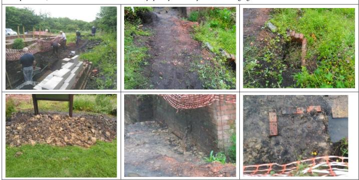
Created a wheelbarrow ramp up the slope to the south of the ventilation fan / winding drum pit, thus making the removal of excavated waste easier. The spoil removed was clay next to the wall, plus cinder ash and some bitumen, it was stacked near the noticeboard. There is a brick square part way along the wall, this requires further investigation.
