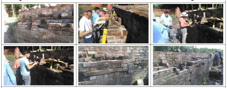
The stabilisation of the east wall of the pit (the engine house side) continued. A lime rich cement mortar was used as the lime helps prevent damage to the bricks and the cement provides the strength. Stabilisation will be the prime focus of the diggers in October as it would be good to finish stabilising the wall before the winter frost.
