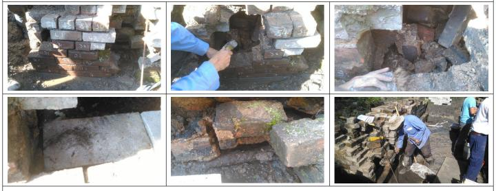
The south west corner of the west wall is being rebuilt as some of the bricks were loose. The bricks were numbered with chalk so that each brick will be replaced in the correct position and orientation during the stabilisation. The bottom left photo shows cement blocks being used inside the hole to strengthen the structure. The bottom middle photo shows the original wood support.
