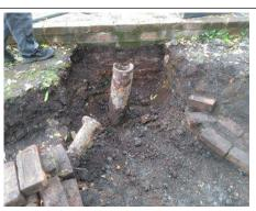
The north western corner of the structure around the old shaft was excavated around the pipes. The excavation expanded when another wall was discovered to the north, this requires further investigation.
