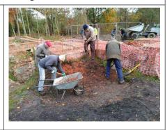
The area to the south of the boiler house and to the side of the chimney was excavated, the material was primarily burnt cinders.
