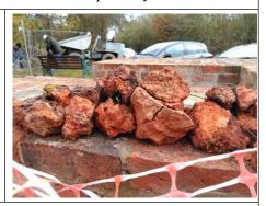
In the corner between the boiler house and chimney were a small number of loose clean bricks that had never been cemented. Some of the material came out in clay lumps.
