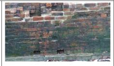
The holes for the engine holding down bolts had been filled with stakes to prevent child sized feet from getting caught. The stakes were replaced with polystyrene blocks. Because the pit to the west of the engine house has been excavated, the pit's holding down bolt holes are now clearly visible from top to bottom, so these can now be used when explaining to visitors.
