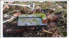
Bit by bit the north wall (next to the fence and hedge) is being exposed, providing evidence of a double thickness brick wall and window ledge cemented in place.
