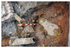
Cast iron pipes since the 18th century were originally horizontally cast but in the 1840s they started vertically or "pit" casting them which made them stronger. It's not easy to tell which ours is, unless we got it grit blasted which is expensive.
