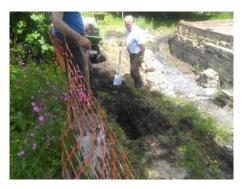
To the west of the engine house and pit activity centred on clearing the top of the tunnel so that the brickwork can be inspected. The power barrow operator takes a rest while the other two fill the barrow, they in turn rest while the spoil is taken away.
