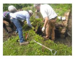
Work continued at the front of the cottage. Cutting through the hawthorn root will at least help kill the stump. One decision is whether to leave the stump in place as an example of what happens when buildings are left to nature, alternatively it could be removed and accept that any damage to the wall would be remedied during consolidation.
