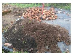
Part of the cleared area next to the cottages was covered with a membrane by Land Management, who also stacked the whole bricks and started the piles of broken bricks and spoil to keep the membrane in place.
