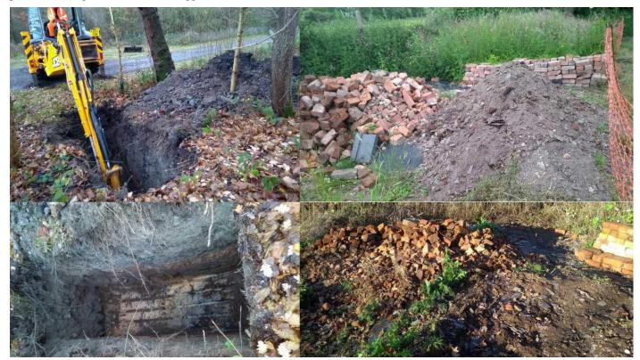
During October a lot of the soil heap was moved to the Coal Authority fenced off area. At the end of November the soakaway / sump was extended and dug down to 2.8m. Trust volunteers have moved the half bricks and slate from the spoil heaps to part fill the sump (now 1m deep at the south end) which has been fenced as it will take several months to fill it.
