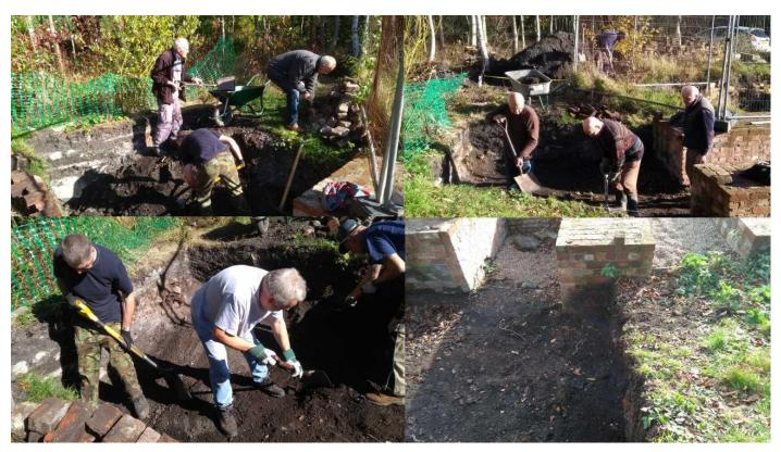
During the two sessions diggers continued excavating the coal stacking pavement outside the largest of the boiler house's three stoke pits. The hole was enlarged to leave room for the proposed sleeper retaining wall. The Trust has agreed that a 1m trench can be dug to both the north and east to find the edge of the pavement. The pavement floor has been reached and found to be in good condition, a thin layer of soil has been left to protect it.
