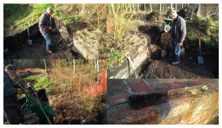
Diggers successfully found the edges of the coal stacking pavement net to the stoke holes. Fortunately there was minimal disruption to the shrub hedge. The vertical metal strip in the earth bank turned out to be a metal stake. Preparations for the retaining walls of wooden sleepers continued.
