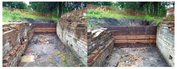
Even on a wet day the sleepers were drying out. The clay between the sleepers and the brick floor will be dug out and stone laid to provide a suitable floor.
