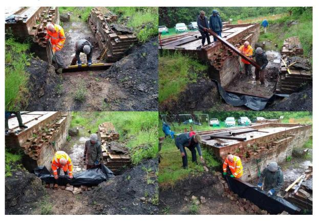
Yes the team did use a spirit level. A plastic sheet was secured to protect the wall from moisture. Bricks behind the sleepers kept them in place and provide drainage.
