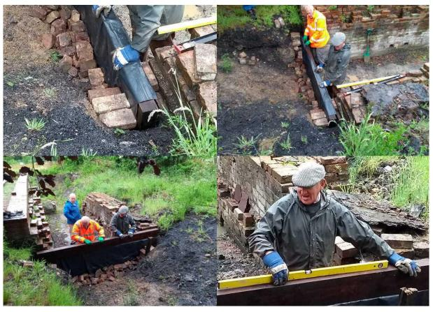
Brick columns at each end kept the sleepers in line. Regular spirit level checks ensured the wall was level.
