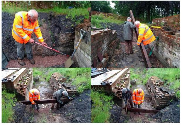
It was a wet morning when the gravel bed was laid. The first of the sleepers required some gentle persuasion to snugly fit into place.
