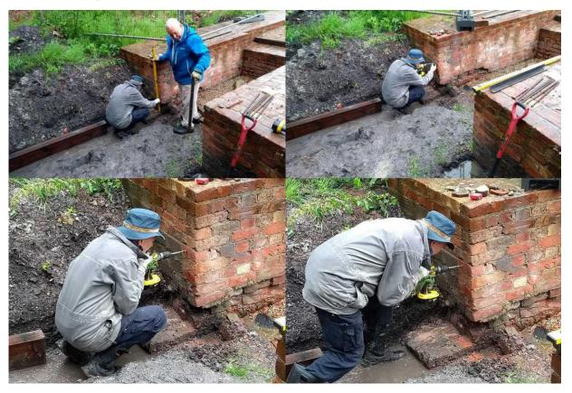
A lot of wet soil had to be shovelled off the coal storage pavement before work on the sleeper wall could start. The focus was on a level baseline and fixing angle iron to the brickwork. Drilling the holes in the bricks required quite a bit of pressure with the drill. Sleepers to be laid in July.
