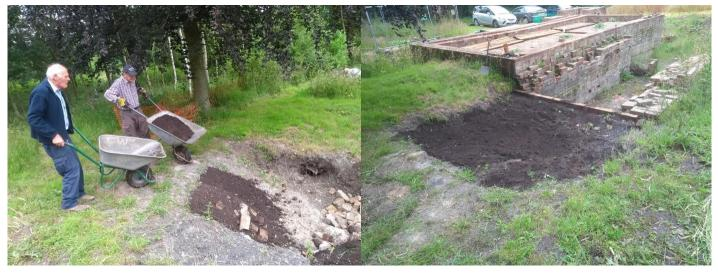
In June the team built the sleeper wall at the north end of the winding drum void, so this month it was filled with spoil previously excavated from the dig. There is now a gentle slope that can be left to settle. The Trust land management team can then finalise the gradient and mow it when the grass appears.
