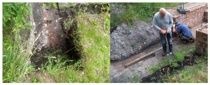
The excavated spur in the coal storage pavement's north west corner was filled with spoil removed from the pavement.
