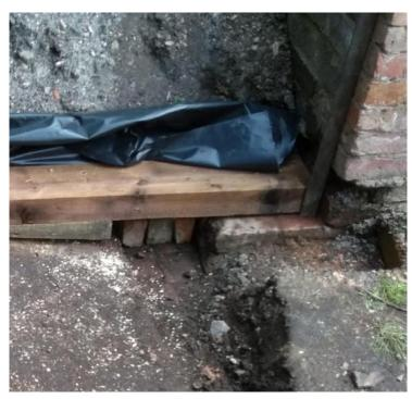
Near where the coal pavement meets the brickwork there is a shallow drain which required the sleeper to be supported by three bricks.
