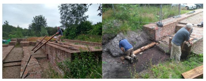
The first three wooden sleepers were moved to the coal storage pavement and carefully fitted in position. It was a slow process getting the levels correct and cutting supports.
