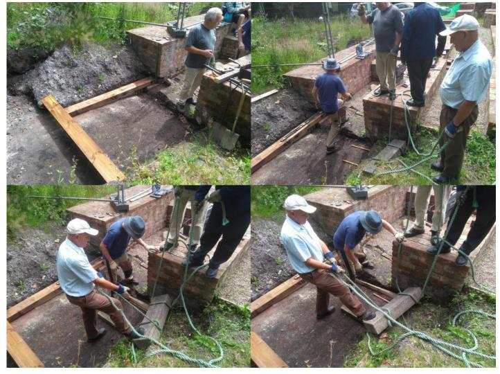
Four diggers used a rope to carefully move the concrete step into position. This method shared the weight, protected the lifters' backs and minimised the risk of trapping fingers and toes.
