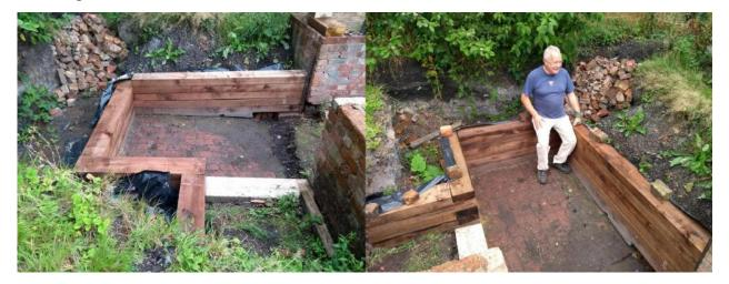
The retaining walls around the section of coal storage pavement that will be displayed are five sleepers high. It is now much easier to envisage the final result.
