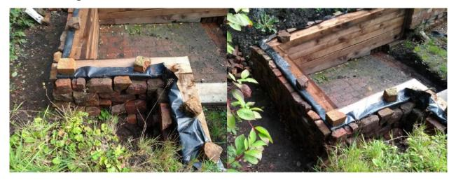
The retaining wall of sleepers was backed by a wall of broken bricks that will help with the drainage.
