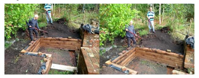
The retaining walls have been back filled with previously excavated material, when complete this will grass over.
