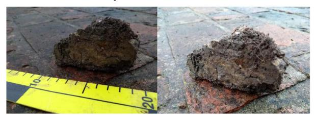
During the dismantling identified triangular clay sections holding the bricks in place.
