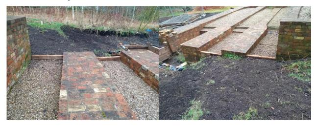
The stoke pits slope had not previously been graded and therefore comprised several multi-directional mini slopes. Retaining sleepers were fitted at the ends of the two filled in stoke pits. These enabled the slope to be dug and raked over to provide a more even gradient that will enable the Trust to maintain the grass.
