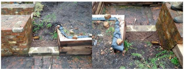
The bottom step had been placed in position to gauge the width when making the sleeper retaining wall. The step was removed then replaced on top of cement to hold it firmly in place. This will provide the foundation for the other steps to be added.
