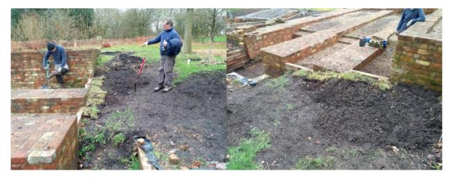
The stoke pit retainer enabled soil and turf to be abutted to it so that a steady slope can lead from next to the engine house to the stoke pit steps.
