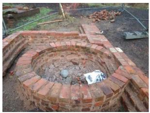
A bricklayer had completed the consolidation of the old shaft and surrounding walls at the turn of the year. This highlighted that the shaft walls had been built as a spiral.
