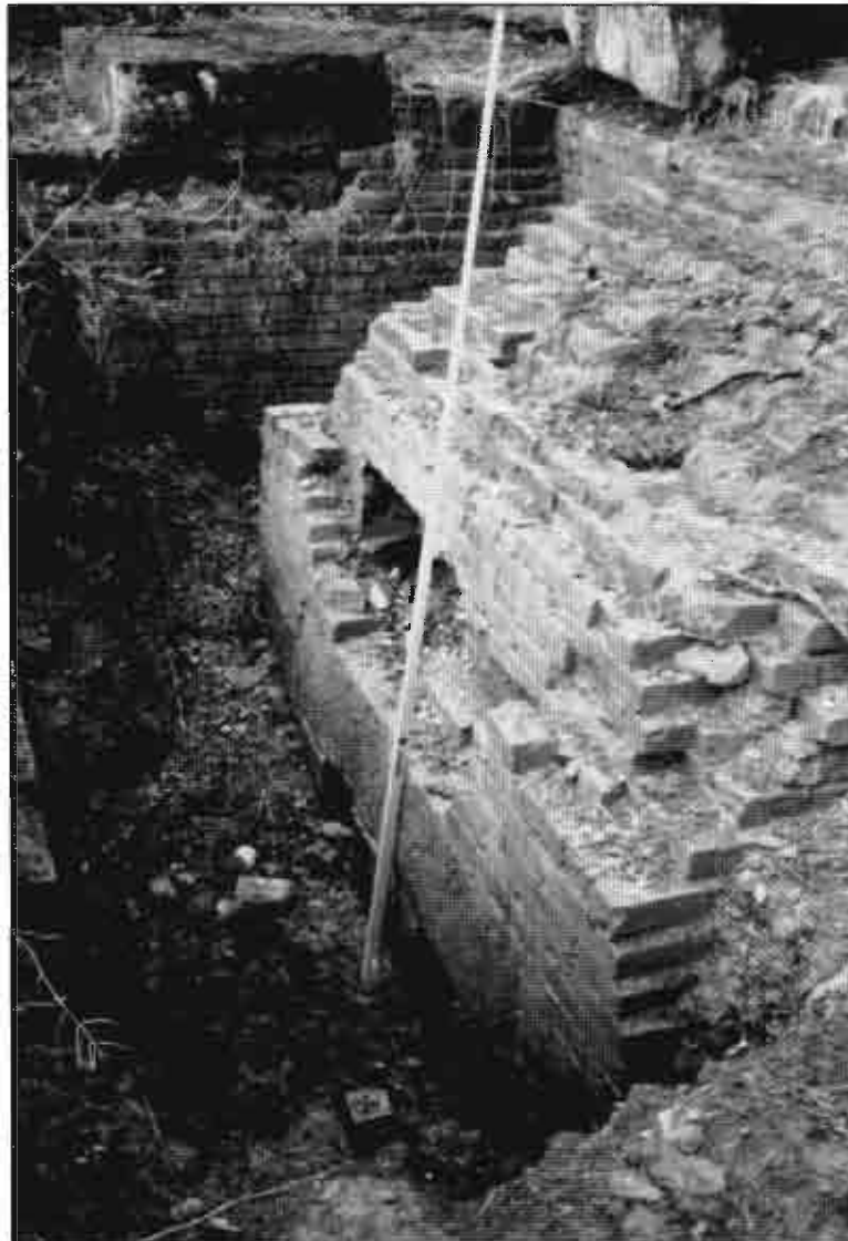
7. The northern plinth in Area 2, showing the badly damaged upper and inner faces. The lower stone block with crow-hole spaces beneath can be seen with Area 1 in the background.
