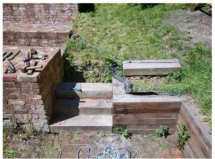
The pieces for the third step were slightly too big, chipping the surplus away was a delicate operation. By the end of the morning the third step up from the stoke pit was in place.
