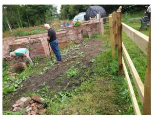
The rebuilding of the well like structure, often referred to as the BBQ, commenced with the most difficult element - getting the head around the pattern of the original construction and working out which bricks fit where.
