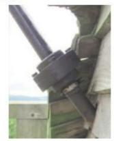
The exterior drive shaft meets the internal drive shaft just outside the cap roof. They were held together by a muff coupling which had failed and was very difficult to remove as it had to be cut off.
