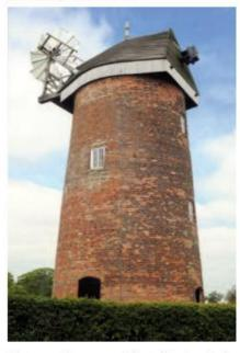
After more than a year of intermittent work, the fantail sails were fully operation and the fantail drive was again turning the cap when the wind changed direction.
