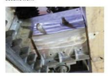
The coach bolts on the pinion shaft lower bearing bracket had sheared or were loose. The team had to fabricate a beam supporting bracket.and fit studs through the wooden beam to hold the bearing in place.
