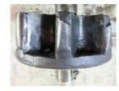
In 2015 the Mill Team noticed that the pinion was damaged. It had only lasted five years. Sadly, they tied off the fantail to stop them turning and removed the curb drive pinion. The team felt that a different engineering solution was needed.
