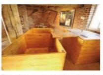
The grain bins and pulpit will be dismantled and moved up a floor. The wall side of the pulpit will have to be modified because the mill is tapered and each floor is smaller than its predecessor.
