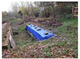
The bricklayer has not returned to point the winding drum wall. To help prevent the frost impacting the unpointed brickwork, the Heritage Trust has covered the wall with a protective sheet.
