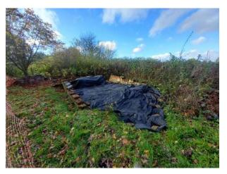
Work continued at the cottages, with the membrane being used to minimise weeds and protect the brickwork from frost.
