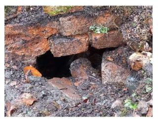
The hole in the tiered brickwork descending from the memorial stones, shows that the brick structure surrounds a large internal hollow.
